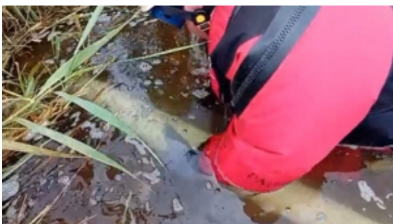
Six layers were applied and smoothed off, curing to form a rock hard, 6mm thick shell around the pipe
