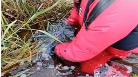
Contractors from SGN entered the river to wrap the gas pipe exposed by scour with SylWrap HD
