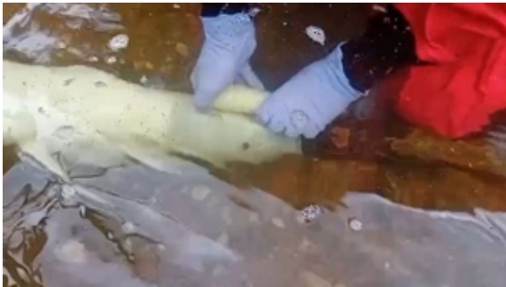
SylWrap HD was wrapped along the length of pipe whilst it remained submerged underwater
