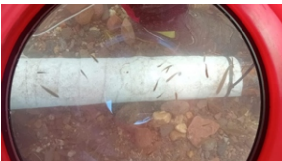
The completed repair left the exposed gas pipe fully protected - and soon began attracting the attention of some intrigued fish
