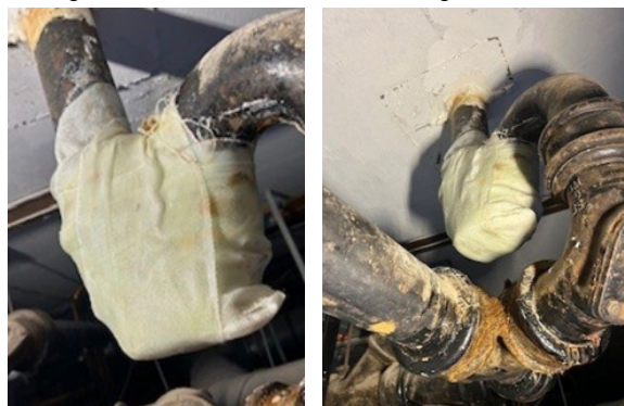
After the leak was sealed with CrackSeal, the U-bend was successfully cocooned with SylWrap HD despite the lack of space and difficult pipe geometry
