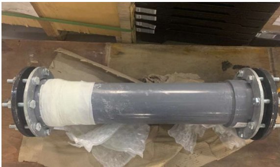
Superfast Aqua PW was applied all around the joint to seal it. SylWrap HD then reinforced a 250mm area of the pipe by creating a thick, robust shell.
