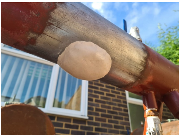
Superfast Aqua PW was formed into a 75mm disc and fixed over the hole
