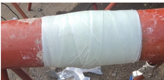
Superfast Aqua PW was formed into a 75mm disc and fixed over the hole
