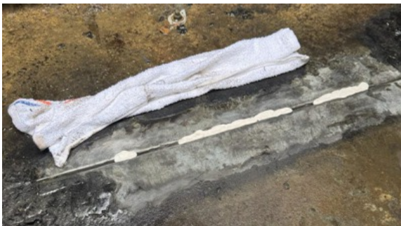
Superfast Aqua PW was forced into the crack, easily adhering to the saturated concrete to seal the leak
