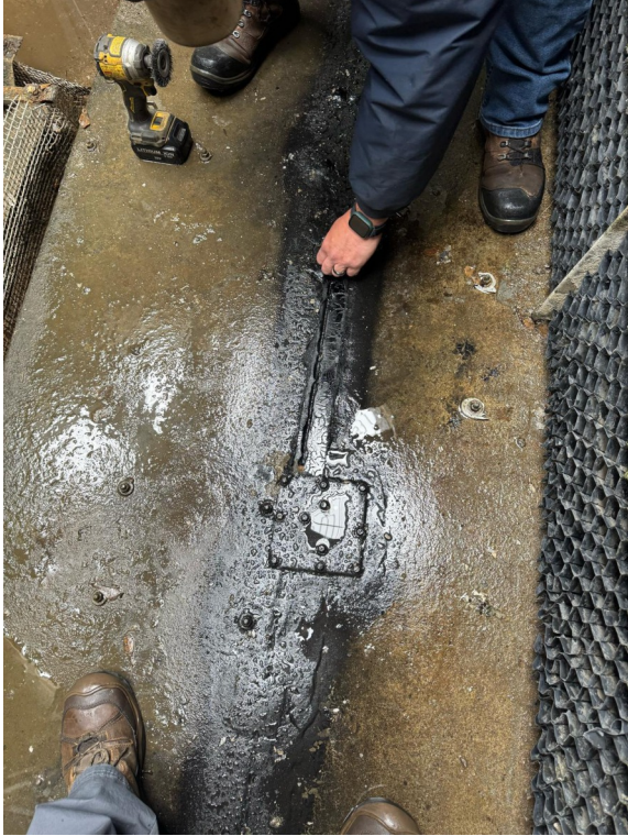
The floor of the cooling tower was leaking through a crack with further damage to the concrete either side
