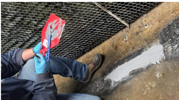
Industrial Metal Rapid rebuilt the floor around the crack where the concrete had crumbled away
