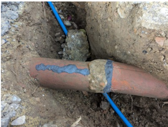
Superfast Steel covered the hairline split across the top of the pipe and was forced into the significant crack next to a junction, almost severe enough to have split the pipe into two separate parts
