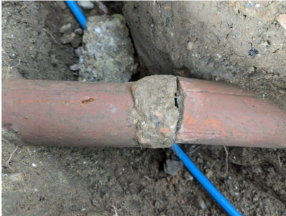
Building work at a UK home had caused ground movement, leading to two cracks to appear in an underground 100mm clay drainage pipe
