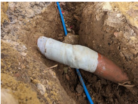
SylWrap HD created a rock hard outer sleeve around the pipe, reinforcing the repair and helping hold the two pieces back together
