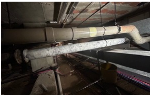
SylWrap provided a rock-hard, impact resistant sleeve across the entire section of cast iron pipe
