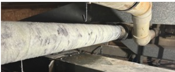
Two SYL633HD SylWrap Bandages were used to reinforce the CrackSeal repair
