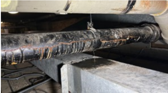
Wastewater was leaking through a 2-metre horizontal crack in the cast iron pipe, located above a ward
