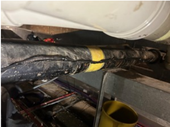
CrackSeal was extruded directly into the crack, hardening inside almost instantly to seal the leak
