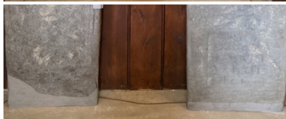
Missing chunks from the bottom of the Dalmally Stones were replaced with a specially manufactured version of AB Original colour-matched to RAL 7037
