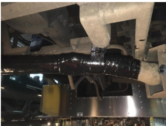
Black-coloured SylWrap HD with inhibitors making the bandage more fire retardant were applied to the conduit pipe, creating an impact resistant shell
