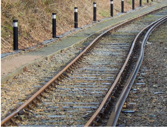
Areas of the UK rail network are powered by a third rail system. Trains take electricity from a conductor line (right of image) on the track bed
