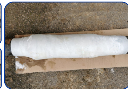
When pressure can be stopped, epoxy putty fills in holes, cracks and missing sections
