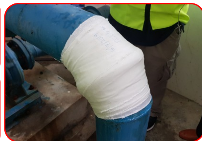
When pressure cannot be stopped, pipe burst tape is wrapped tightly around the leak area
