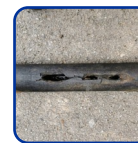
When pressure cannot be stopped, pipe burst tape is wrapped tightly around the leak area
