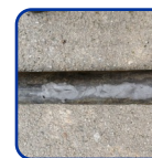
When pressure can be stopped, epoxy putty fills in holes, cracks and missing sections
