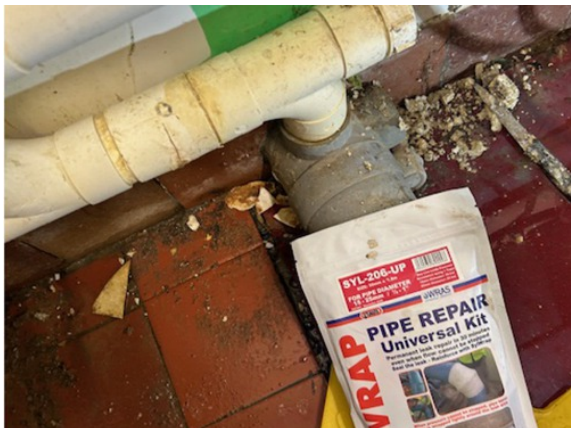
The golf club called their drainage contractor, who kept a stock of Sylmasta product on his van - including a SylWrap Universal Pipe Repair Kit
