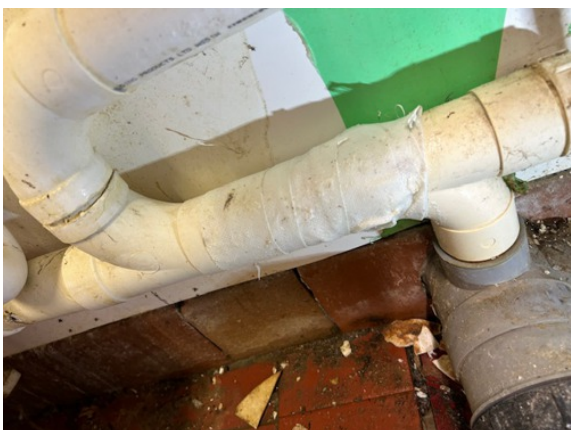
Wrap & Seal was wrapped around the split, sealing the leak. The repair was then completed with application of SylWrap HD to provide a rock-hard, impact resistant layer of protection
