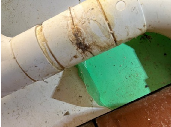
A 50mm plastic drain pipe connected to the back of the dishwasher was found to have a split around its entire diameter, leaking water all over the kitchen
