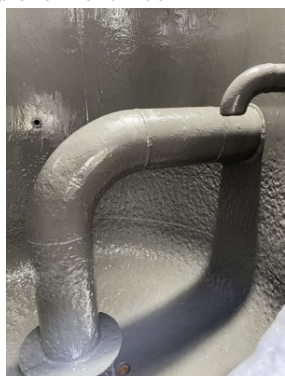
Liquid Metal repaired the heavily corroded metalwork inside the heat exchanger plenum chamber
