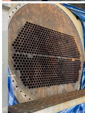
Worn tubes inside the chamber and the condenser faceplate were also refurbished with Liquid Metal
