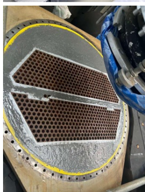
Worn tubes inside the chamber and the condenser faceplate were also refurbished with Liquid Metal
