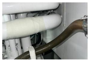
Wrap & Seal sealed the leak with pressure resistance to 2 bar, followed by overwrapping with SylWrap HD for reinforcement and protection
