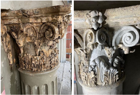
Each damaged column top - known as a capital - was thoroughly cleaned before undergoing repair
