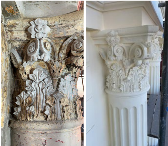
AB Original was carved to replace missing details before the entire facade was painted white
