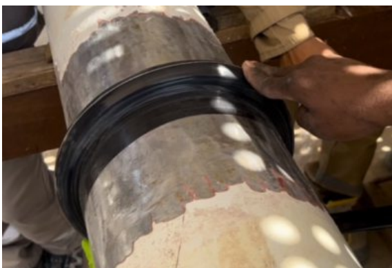
Multiple Wrap & Seal applied to leaking welding joints built repairs capable of holding 10 bar pressure
