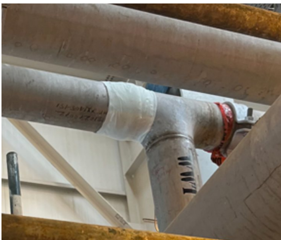
Repairs were reinforced with SylWrap HD, including to difficult-to-access sections of overhead pipe
