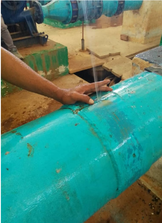
Water had been escaping the 300mm steel pipe for two weeks through a 4mm hole at 6 bar pressure
