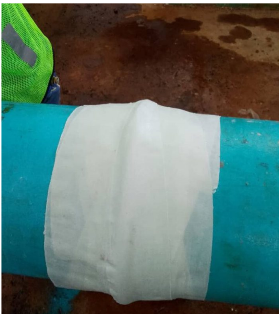
Three 50mm x 11m Wrap & Seals built a repair with enough resistance to withstand 6 bar pressure, followed by reinforcement with SylWrap HD
