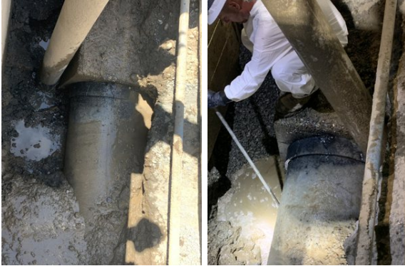
The break was somewhere beneath the joint in the pipe at the point it passed into the concrete wall
