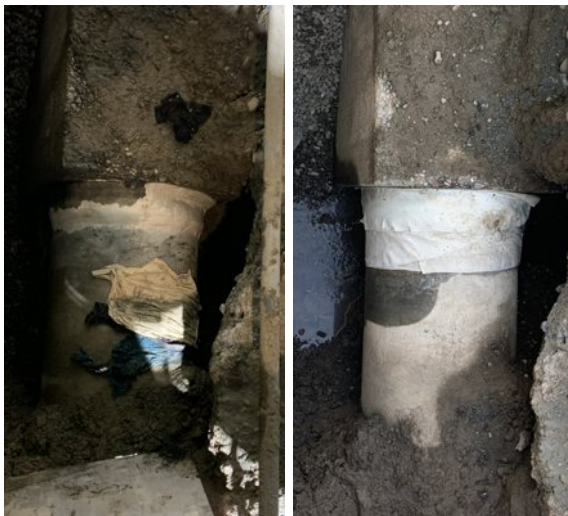
Once water loss had been reduced to an acceptable level by encompassing the leak area, the repair was reinforced with SylWrap HD Bandage
