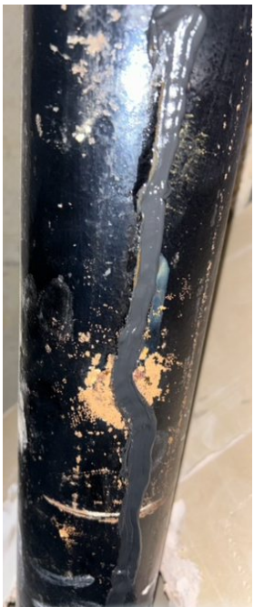
The crack was sealed by extruding CrackSeal directly into it. The entire length of pipe was then reinforced with SylWrap HD for a permanent repair
