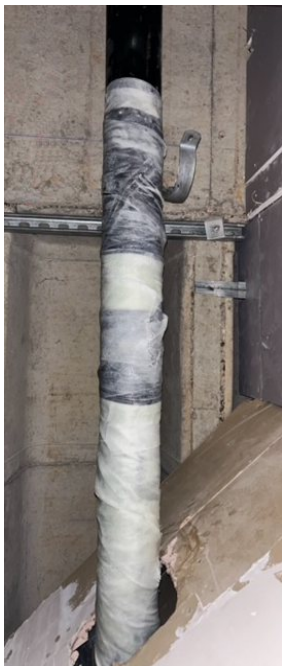
The crack was sealed by extruding CrackSeal directly into it. The entire length of pipe was then reinforced with SylWrap HD for a permanent repair
