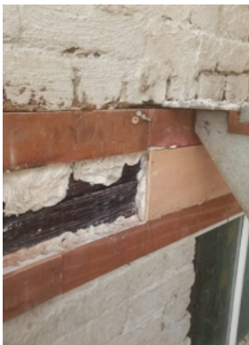
The repair created a flat, smooth surface which could be rendered onto directly
