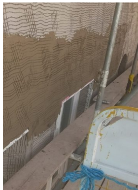
The repair created a flat, smooth surface which could be rendered onto directly
