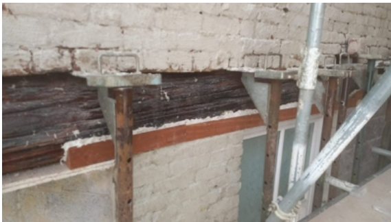
Hardwood inserts were bonded to the AB Original in areas where voids were particularly deep, helping to reduce the amount of putty needed for the application
