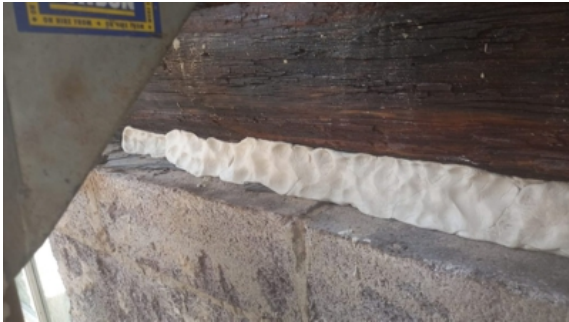
AB Original was pushed into all gaps in the wooden beam left by rotting, permanently filling the damage
