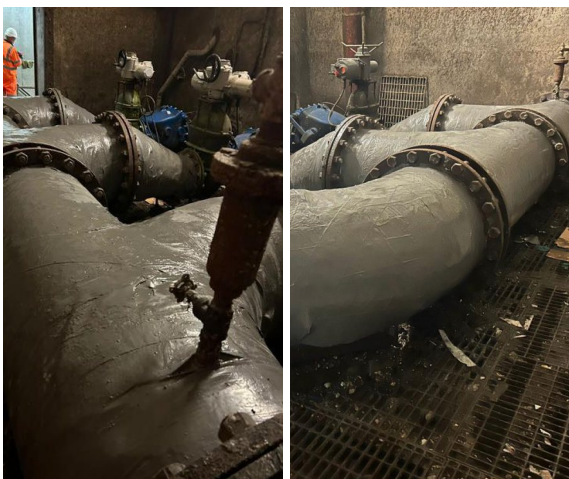
Liquid Metal and SylWrap HD combined to form a robust outer shield protecting against corrosion
