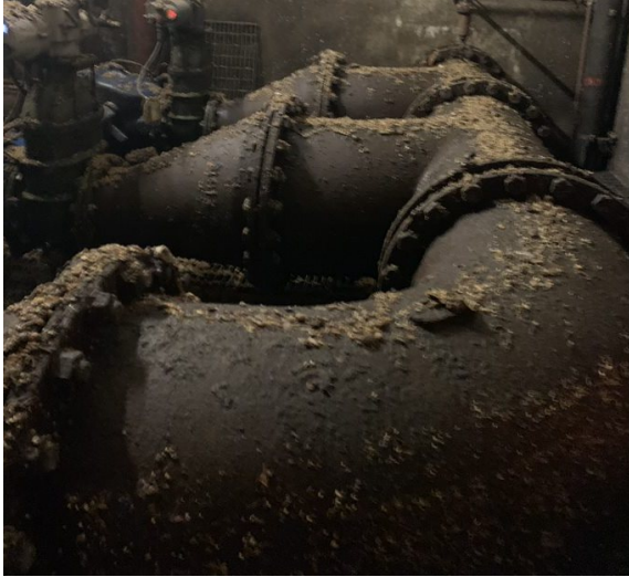
The pipe system was covered in contaminants and showing early signs of external surface damage
