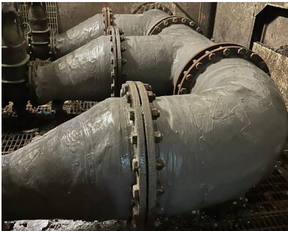
The pipe system was covered in contaminants and showing early signs of external surface damage
