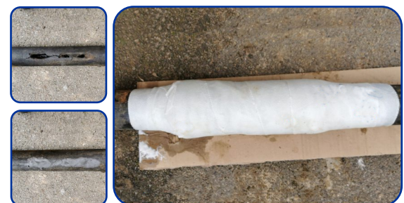
When pressure can be stopped, epoxy putty fills in holes, cracks and missing sections
