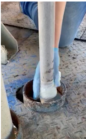
The repair was reinforced and protected with SylWrap HD Pipe Repair Bandage
