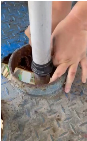
Wrap & Seal Pipe Burst Tape sealed the live leak despite the space constraints around the pipe
