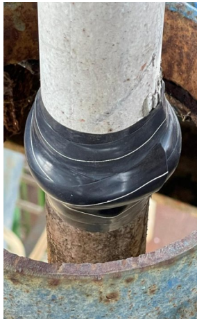
Wrap & Seal Pipe Burst Tape sealed the live leak despite the space constraints around the pipe
