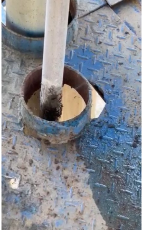
Alcohol juice was spraying through a pinhole leak at a point where the line passed through a circular hole in the upper floor of a platform
