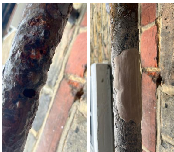
Superfast Aqua PW sealed holes in where corrosion had breached the line in several places
