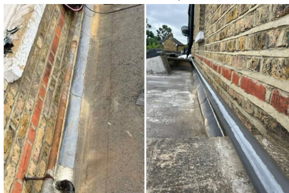
Superfast Aqua PW sealed holes in where corrosion had breached the line in several places
