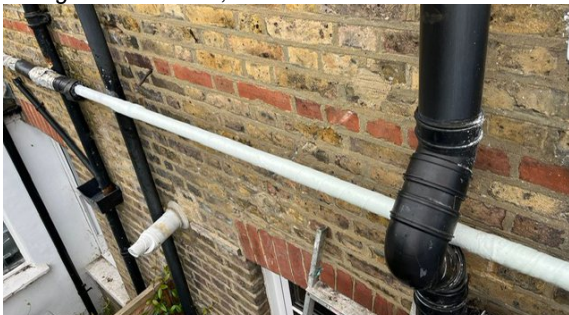
SylWrap HD was applied over the Liquid Metal coating, forming an impact resistant shell
