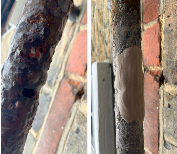
Superfast Aqua PW sealed holes where corrosion had breached the pipe in multiple places
