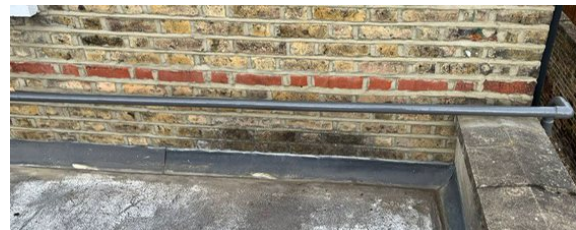
The pipe was painted in Liquid Metal to reinforce and strengthen the brittle, corroded metalwork
