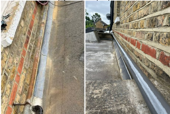
Superfast Aqua PW sealed holes where corrosion had breached the pipe in multiple places
