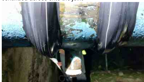
Once the joint ends had been encapsulated, Wrap & Seal was applied directly over the leak to create a ridge increasing the pressure resistance of the repair
