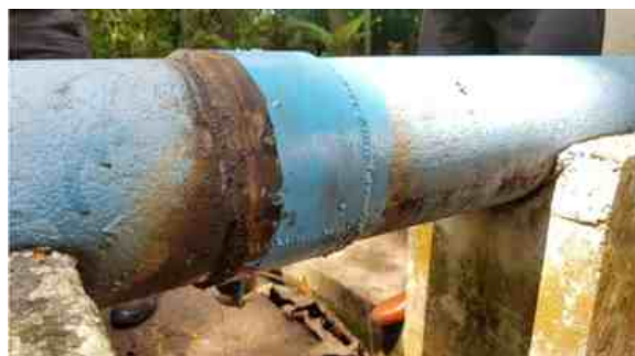
Water was seeping from both ends of the saddle joint, one of which was suffering from heavy corrosion
