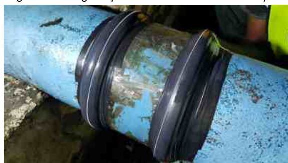
Wrap & Seal was applied to both ends of the saddle joint, successfully sealing the pipe
