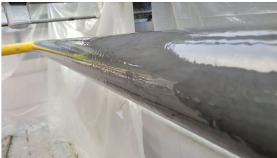
Rust, grime and paint were ground off the pipe and the three metre section coated in Liquid Metal
