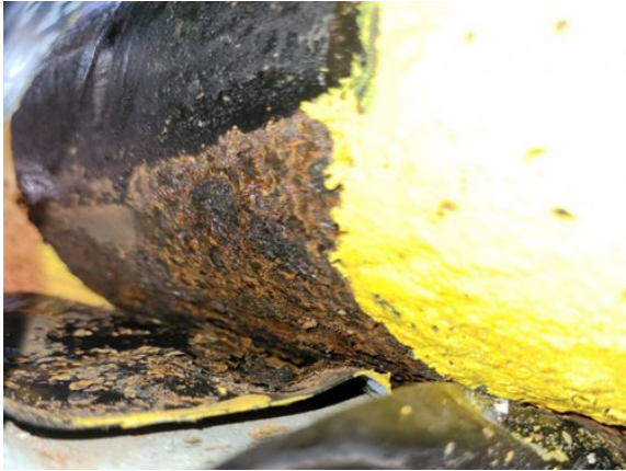
The pipe was heavily corroded where water had been trapped between a protective PVC tape and the line
