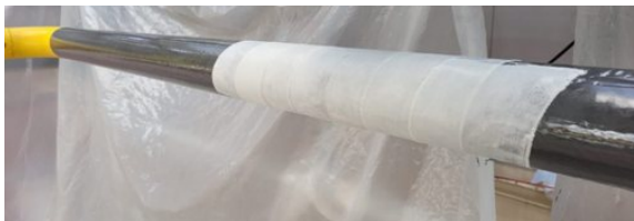
SylWrap HD increased the thickness of the weakened area where the pipe had contact with the U-support
