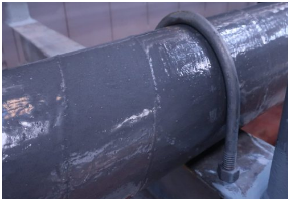
A second Liquid Metal coating was applied over SylWrap HD and the pipe fixed to the U-support
