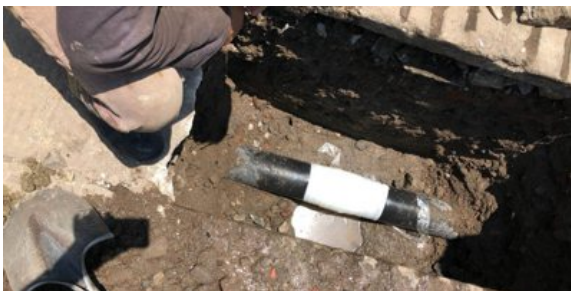
After the leak was sealed with Wrap & Seal, SylWrap HD Bandage replaced the protective concrete coating
