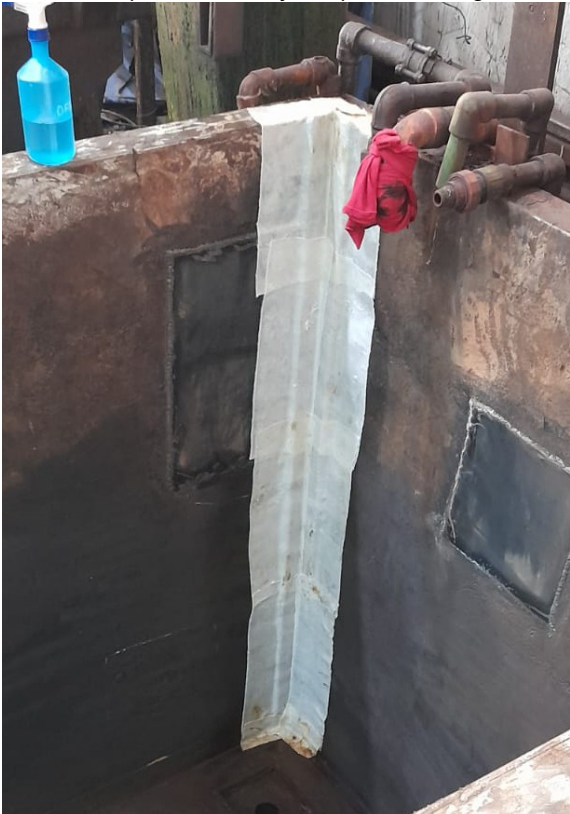
Patches of SylWrap HD pressed and smoothed over each corner created a watertight seal between the weld and the existing iron frame of the tank
