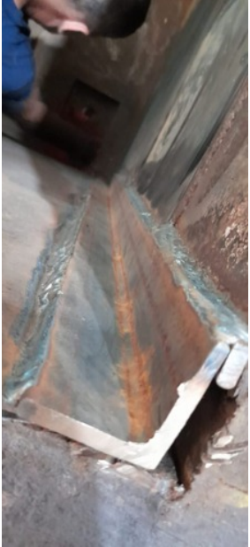
New metal corners were welded to reinforce all four corners of the chromic acid tank. These corners were then encompassed with SylWrap HD Bandage
