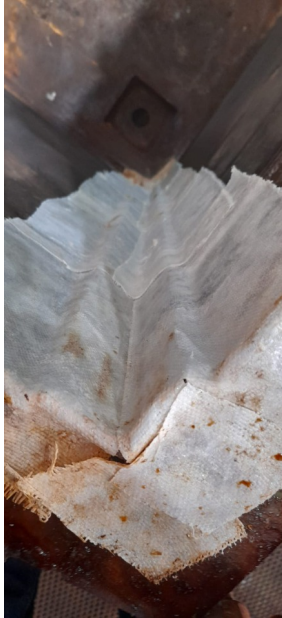
New metal corners were welded to reinforce all four corners of the chromic acid tank. These corners were then encompassed with SylWrap HD Bandage
