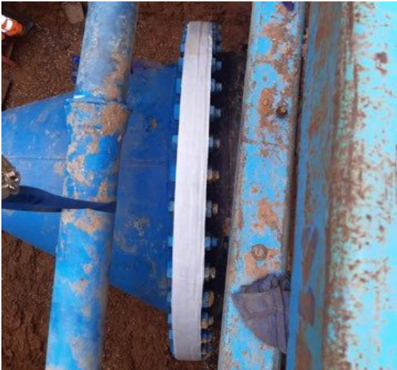
Wrap & Seal was applied all around the flange to seal the leak. It was then overwrapped with SylWrap Pipe Repair Bandage
