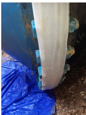
A SYL412HD Bandage was the perfect 100mm width to wrap around the flange, curing to form a rock-hard shell which tree roots would not be able to penetrate in future
