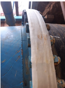
A SYL412HD Bandage was the perfect 100mm width to wrap around the flange, curing to form a rock-hard shell which tree roots would not be able to penetrate in future
