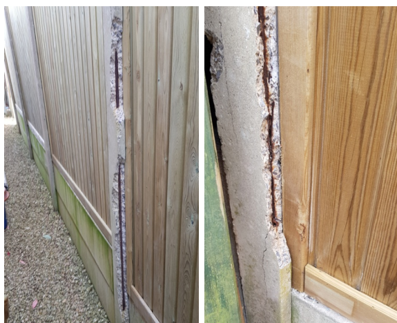
Concrete cancer had caused serious damage to the fence posts, worsened when the posts were disturbed during the installation of the new trellis
