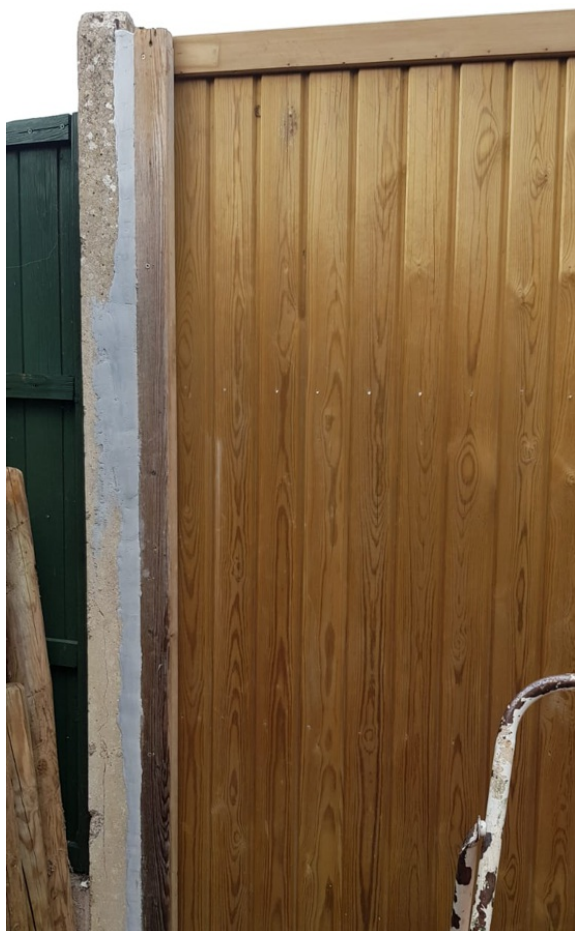
Sylmasta AB filled in all the damage in every fence post whilst also offering protection against corrosion to the inner steel rods
