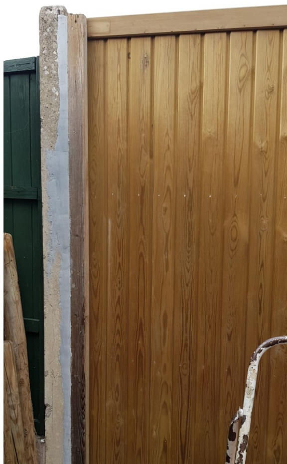
AB Original filled in all the damage in every fence post, whilst also offering protection to the inner steel rods against future corrosion
