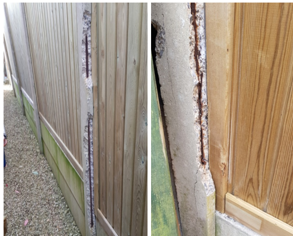
Concrete cancer had caused serious damage to the fence posts, worsened when they were disturbed during the installation of the new trellis
