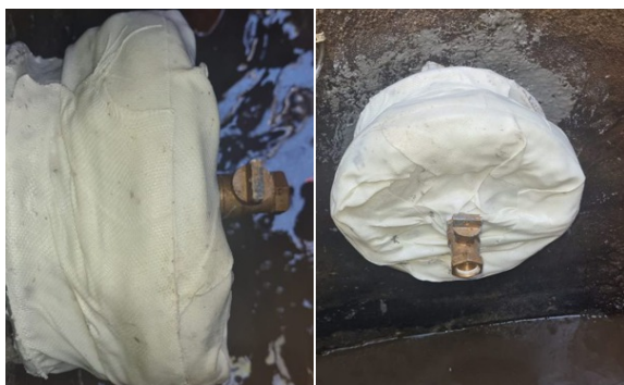
SylWrap HD was wrapped around the stub and smothered over the flange plate for protection
