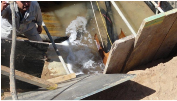
The line was isolated, excavated and re-pressurised. So much water escaped that the hole dug to access the pipe became instantly flooded
