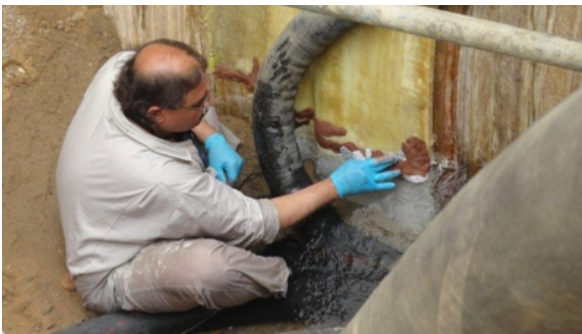
Superfast Copper sealed smaller holes in the line
