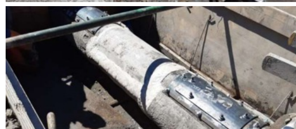
AB Original encapsulated the clamp, sealing all areas which the pipe was leaking from
