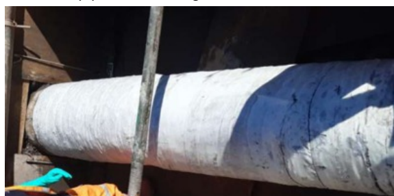
SylWrap HD Bandage was wrapped across the entire length of the pipe, completing the repair
