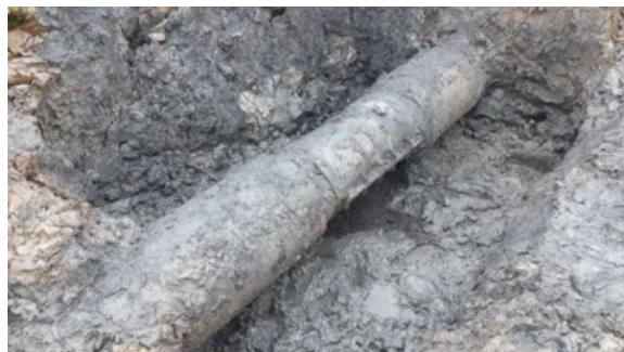
The leaking pipe ran beneath salt marshes, leaving an eight hour window with the tide out to access, excavate and clean the pipe, and seal the leak
