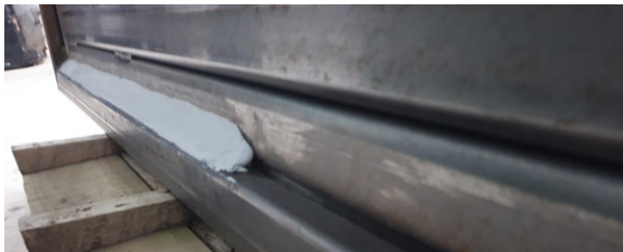
A strong steel frame was built for the replacement gates, onto which wooden slats would be fitted
