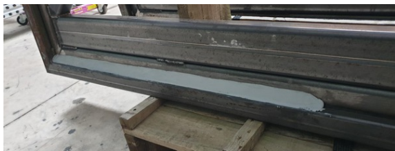
AB Original was formed into a bevelled edge to create a run-off preventing water pooling at the base of the frame and rotting the slats
