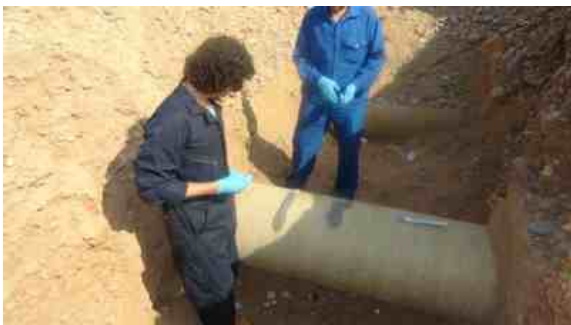
The completed repair with all damaged areas filled in. After completion, the pipe was buried again
