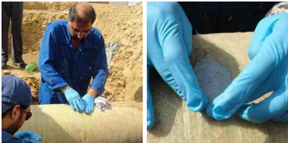
Superfast Steel was pushed onto the pipe to fill the imperfections and rebuild the thickness of the outer line where it had weakened
