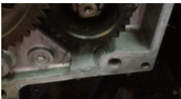
Completed repair with crack seamlessly filled in
