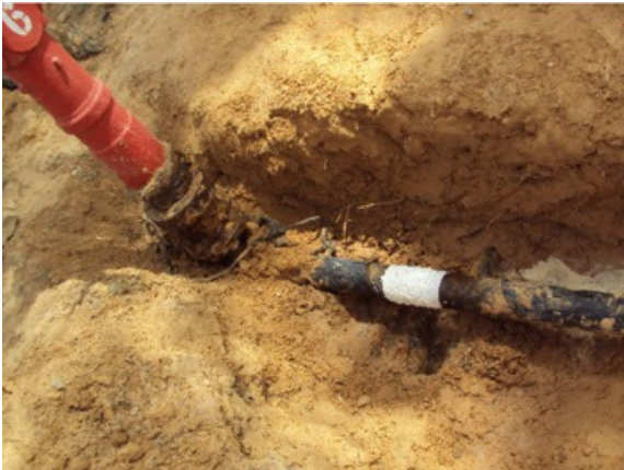
A trench was dug with enough clearance to reach the below-ground section of pipe. It was then repaired using Wrap & Seal and SylWrap HD Bandage
