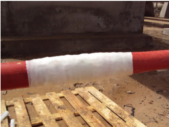
The above-ground section was successfully sealed using Wrap & Seal and then further protected with SylWrap HD Pipe Repair Bandage
