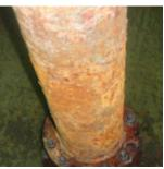
Lower sections of the pipe were badly corroded
