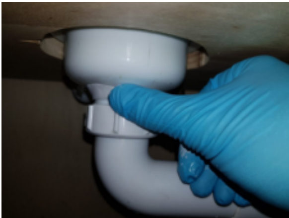
Superfast Plastic was kneaded by hand, formed into a sausage shape and pushed over the cracks in the pipe whilst the putty remained soft
