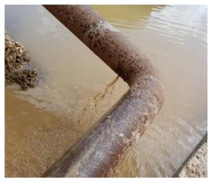
The 150mm steel pipe was leaking from a pinhole close to a 90 degree elbow bend, meaning that a pipe repair clamp would not be effective
