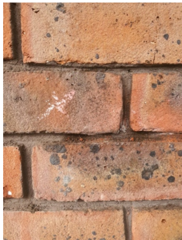
AB Original mixed with brick dust created a seamless repair with the brick
