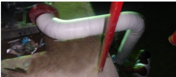
Completed reinforcement of the upper section of pipe
