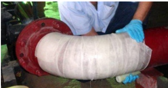
SylWrap HD applied to one of the elbow bends
