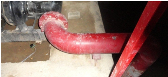
There were two elbow bends in the line, providing a difficult geometry for wrapping around
