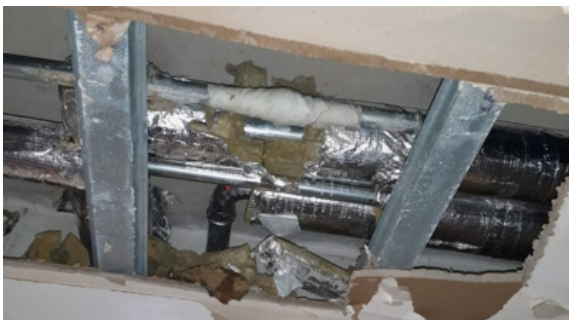
SylWrap HD reinforced the repair by creating a rock hard layer around the entire section of pipe
