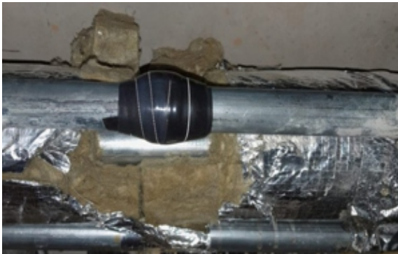
Wrap & Seal formed a solid rubber band over the leak
