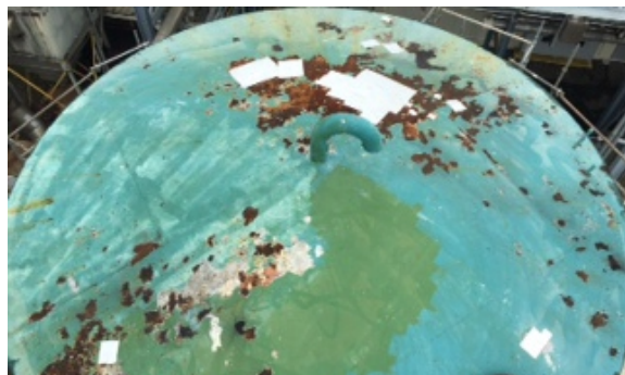
E190 Brushable Epoxy Resin was coated onto strips of Fibreglass Tape to patch repair the holes
