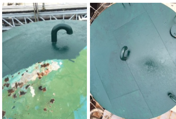
Three layers of Ceramic Brushable were painted onto the patched roof, creating a new outer surface with resistance to corrosion and abrasion
