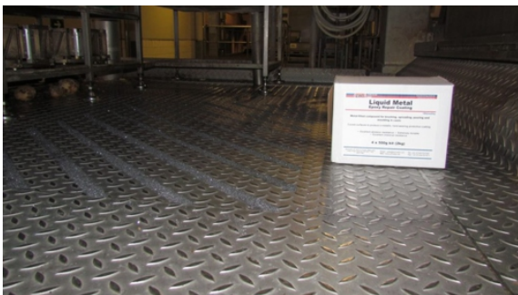
Liquid Metal was painted onto the surface in strips created using masking tape. Silicon carbide grit was then sprinkled over the top whilst the coating remained tacky
