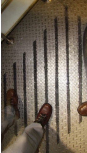
Existing anti slip surfaces had become worn and ineffective. These needed to be replaced, as well as new surfaces installed in other areas
