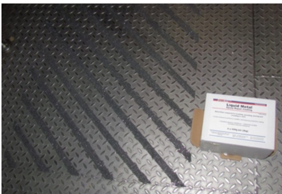
Once Liquid Metal cured, it left the grit permanently bonded to the flooring. This created a robust anti slip surface
