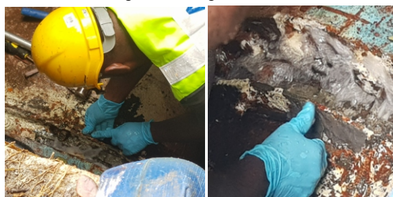
Superfast Steel filled the cracks in the pipe, fixed plastic plug in place and encompassed the flange
