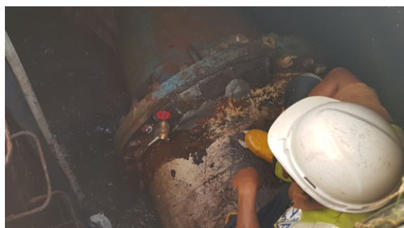
A tap was fitted to the valve, containing the final leak and completing the 'impossible' repair
