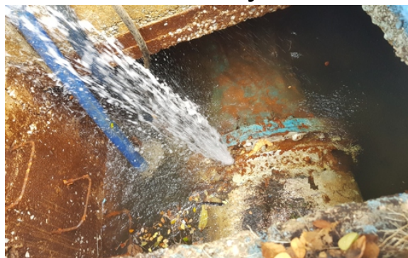
Pressurised water was escaping multiple cracks in the main, flooding the underground chamber
