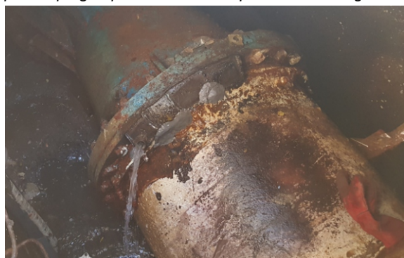
A valve fitting was fixed in place with Superfast Steel, channelling the final leak path through the valve
