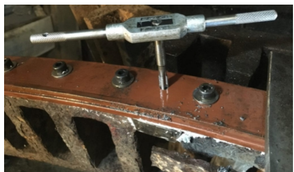
Hoop screwed into the wheel to complete repair
