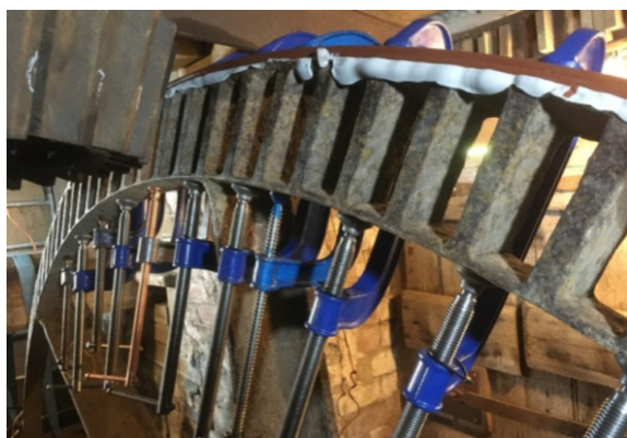
Clamps held the steel hoop in place whilst AB cured
