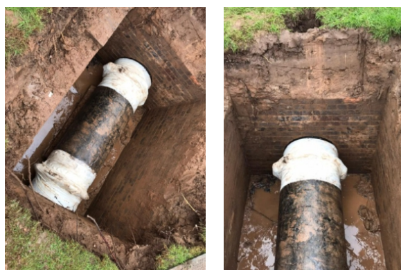
Completed repair prior to reburial of the pipe
