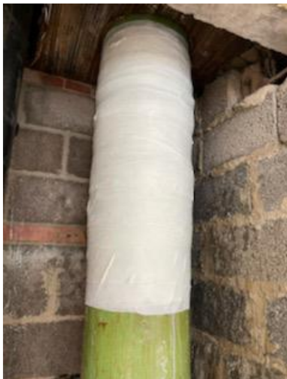
Two SylWrap HD Bandages completed the repair
