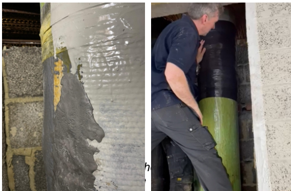
Superfast Steel and Wrap & Seal used to seal the leak
